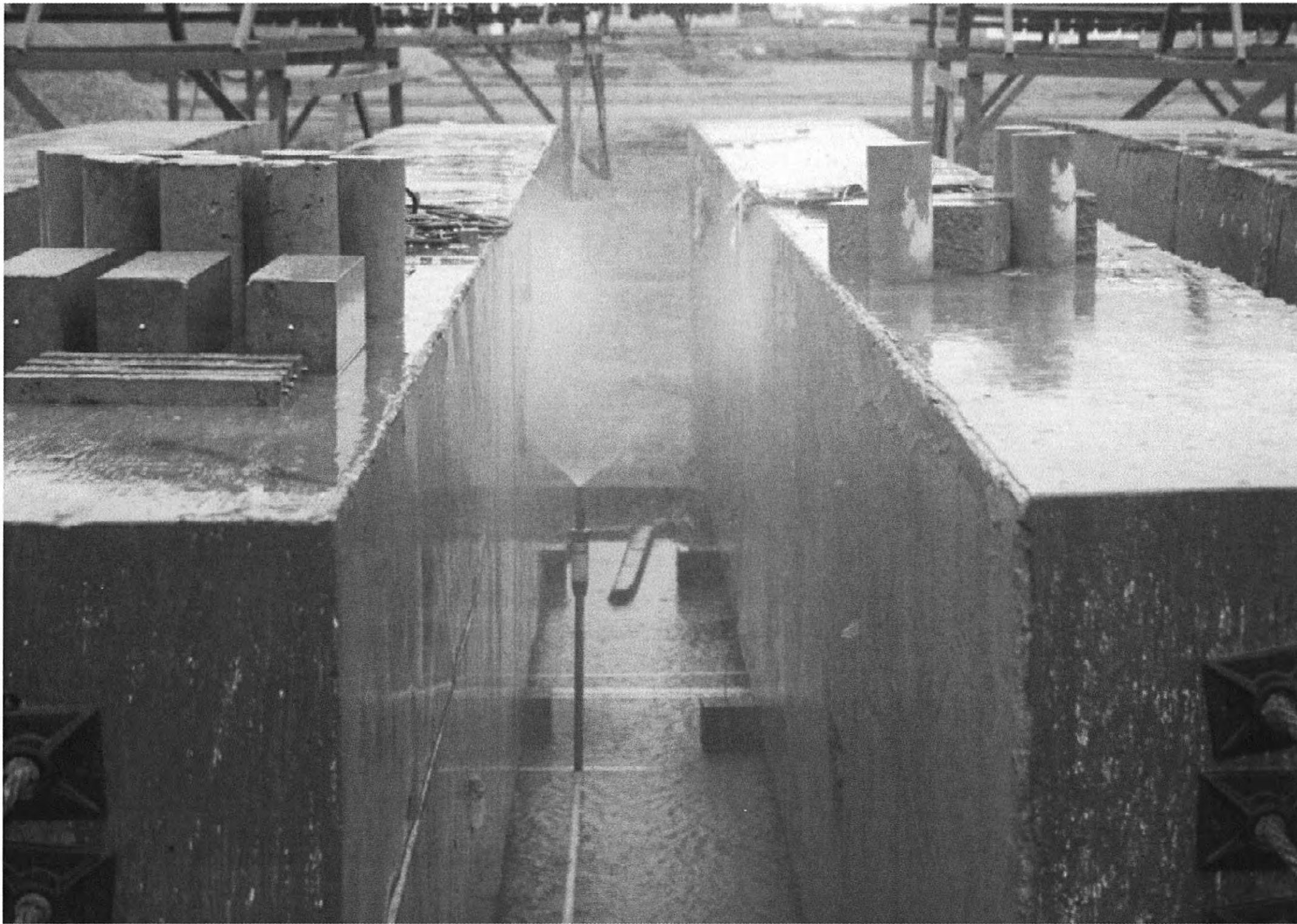
Figure 3-4. Sprinkler System between Two LSC Specimens.
