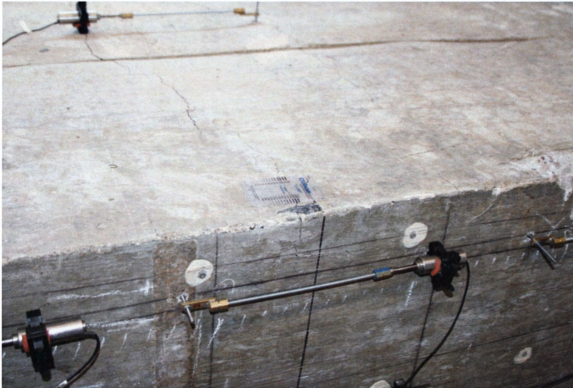
Figure 5-43. Flexural Crack above the Center Support from Three-Point Test (LSC5).
