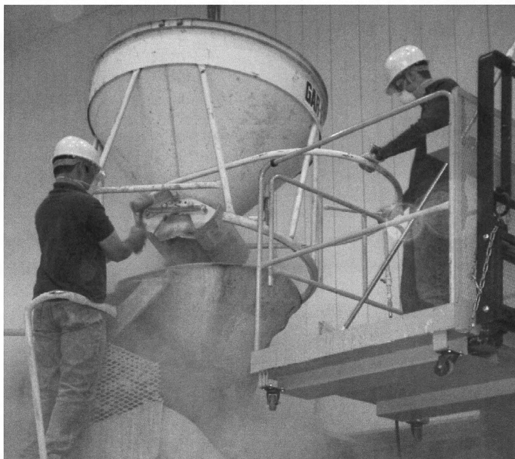
Figure 2-19. Dumping Cement into the Mixer.
