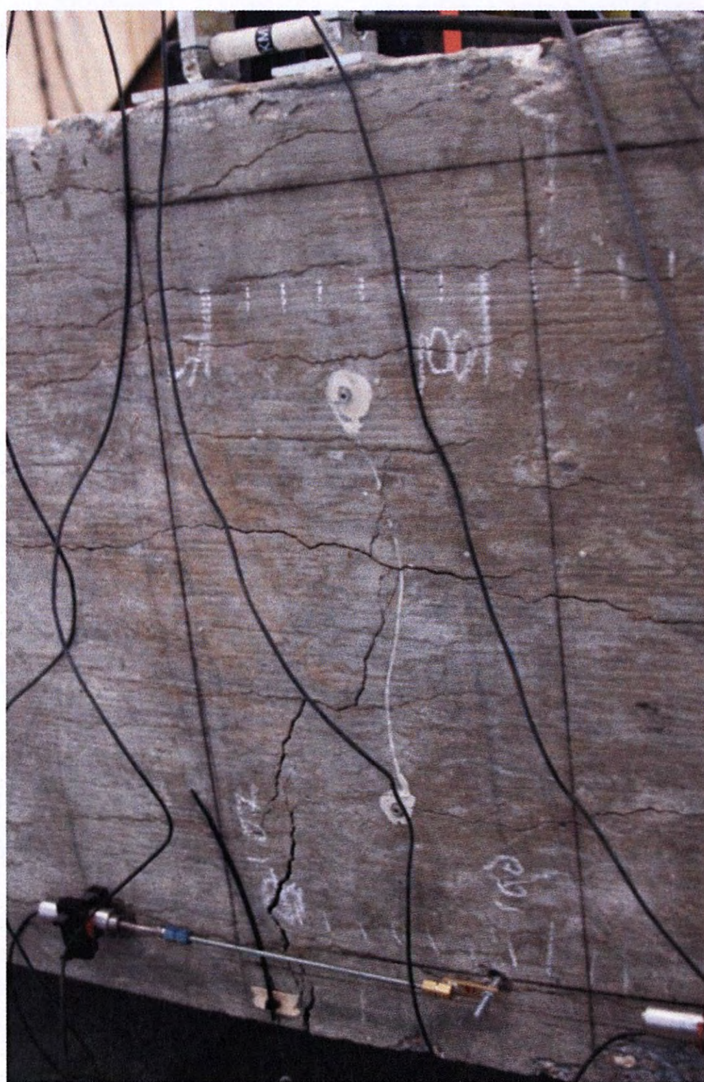
Figure 5-31. Flexural Crack under Actuator 1 during the Four-Point Test for LSC5.
