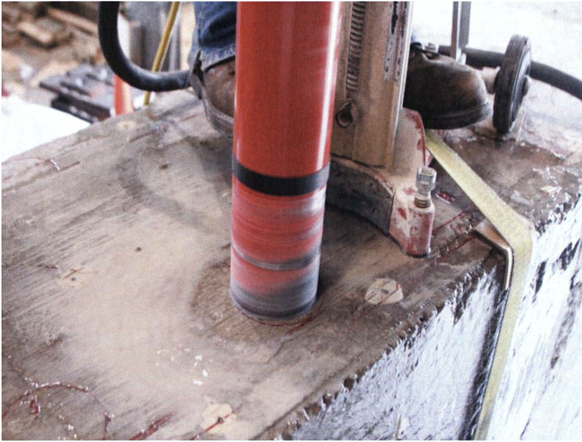
Figure 3-27. Coring Machine Attached to Beam.
