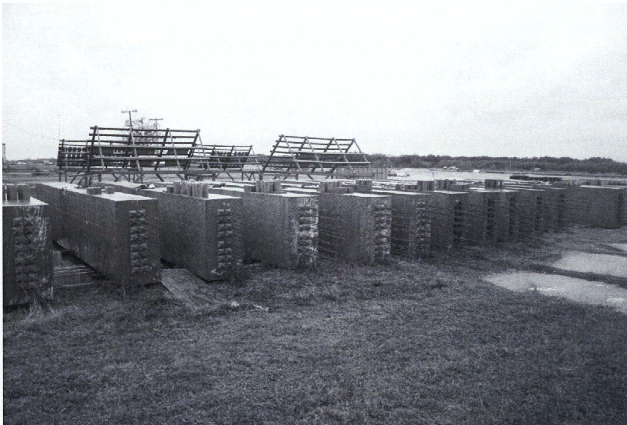
Figure 3-3. LSC Specimens Exposed to the Environment at the Riverside Campus.
