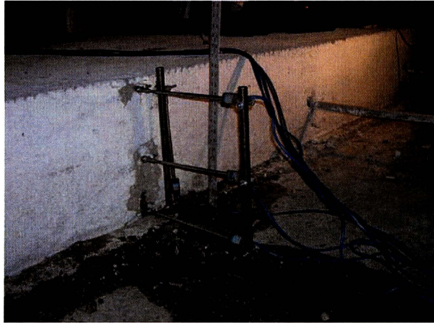
(a) Crackmeter for transverse movement measurements
