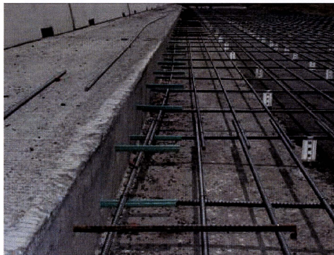
Figure 2.2: Tied and doweled sections
