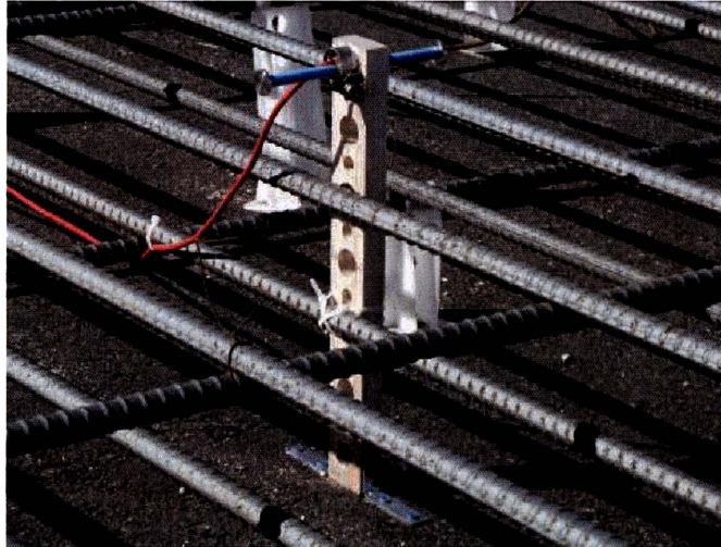
(a) VWSG installed with a chair
