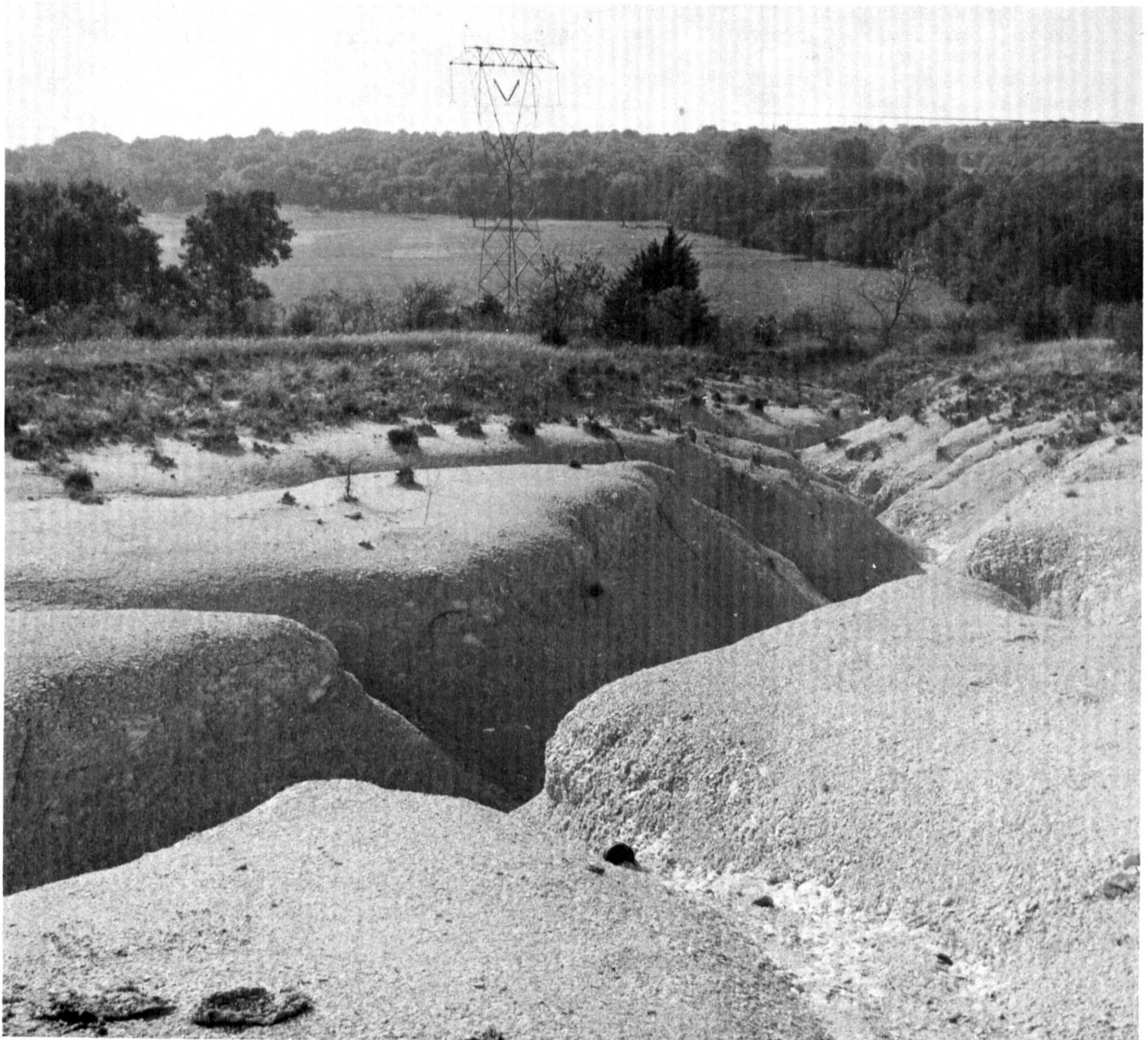
Figure 12.—Area of Whitewright-Gullied land complex showing large bare area of chalk extending from edges of gully.
